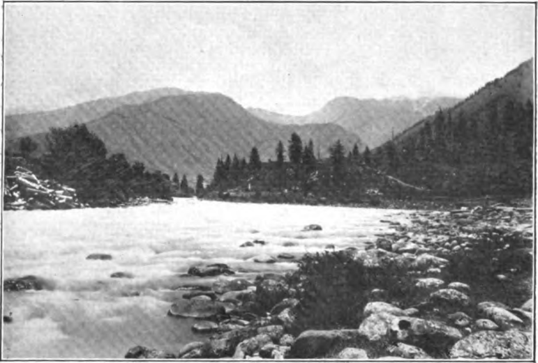
Logs ready to be floated down stream
