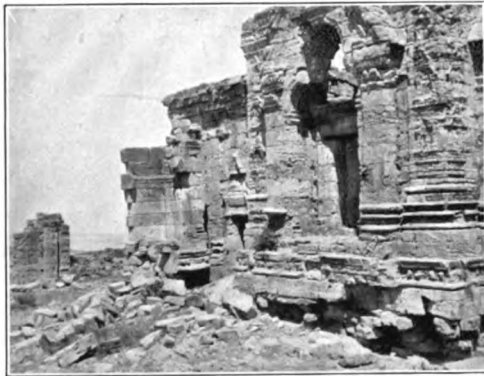
Grand entrance turned to the west
