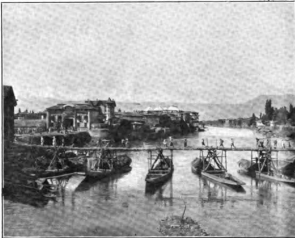
Rebuilding bridge after floods, 1898
